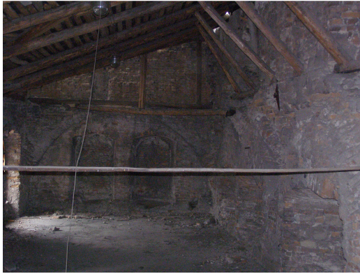
Fig. 34. Temporary roof over the western synagogue's body: photo taken in 2008.
