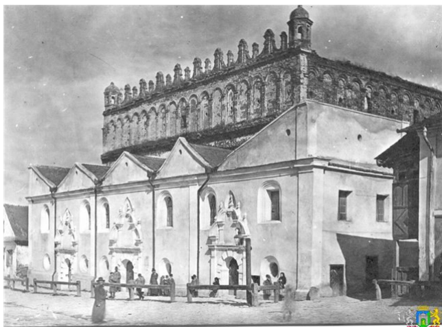
Fig. 27. Synagogue in Zhovkva before the restoration carried out in 1908: photo taken in the early 20th century. Lviv Historical Museum.
